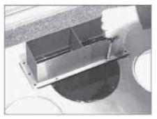
3. Mount the 3-1/4"x10" starting collar on top of transition piece with remaining screws.
